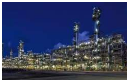
Fig.5. Industrial and Midstream | Source: https://www.galp.com/corp/pt/media/comunicados-ofpress-release/press-release/id/882/refinery-of-Sines-celebrate-40-years-with-new-vacancy-of-investments
