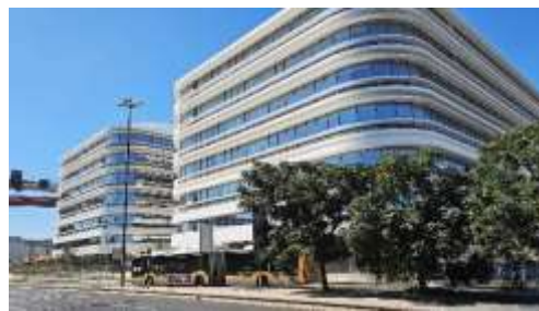
Fig. 2. Alcântara Lisbon Offices| https://www.facal.pt/en/noticias/alcantara-Lisbon-offices-hello-knife/
