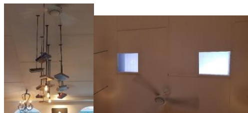
Figure 17. Ceilings at Nadhi Heritage
