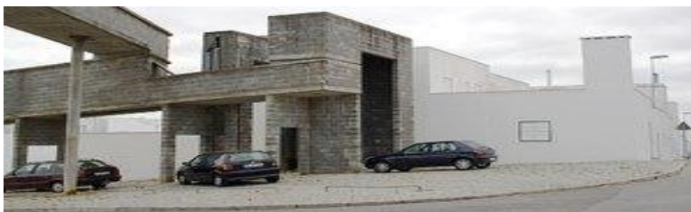
Figure 148: Siza Vieira, Quinta da Malagueira Social Housing, View of the aqueduct. Source: http://media.archinform.net/m/70033064.jpg The concrete blocks are a simple material with a strong truthful presence, and provided an inexpensive solution for the aqueduct which has various axes in the configuration space that will be built. They have, for example, gelled together the housing structures which surround the aqueduct, allowing for an element with a very strong presence to give unity and continuity to the development,
