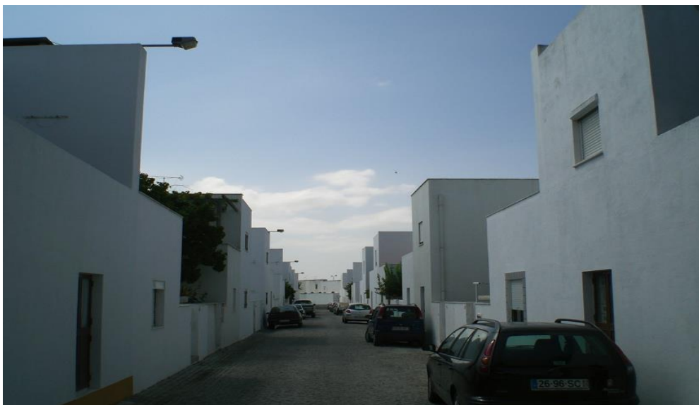
Figure 154: Siza Vieira, Quinta da Malagueira Social Housing. Source: Photograph by the author.
