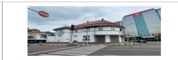
Figure 2: Current Pencil Building Source: author's documentation
