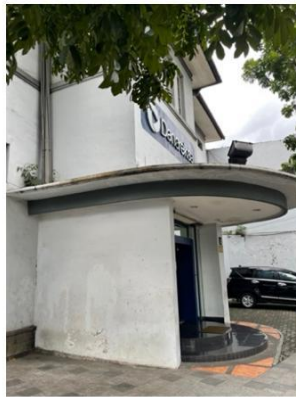
Figure 5: Entrance into The Pencil Building Source: author's documentation
