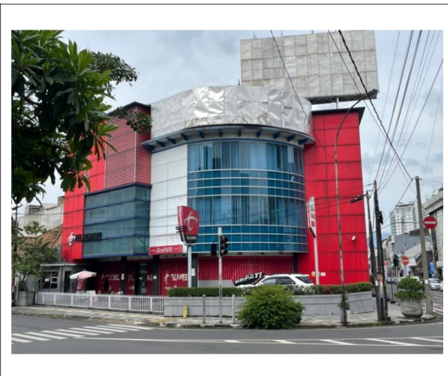
Figure 20: The Grapari Telkomsel Building Source: author's documentation
