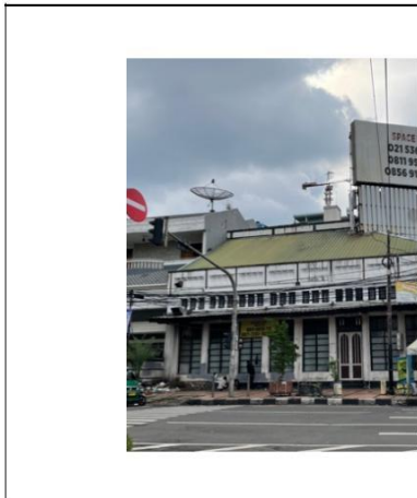
Figure 11: Asbestos Roof of The Vigano Building Source: author's documentation
