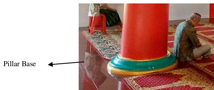
Figure 14. Pillar base inside the Cheng Hoo Purbalingga Mosque (Source: Documentation of Imam Ramadhan, 2017)
