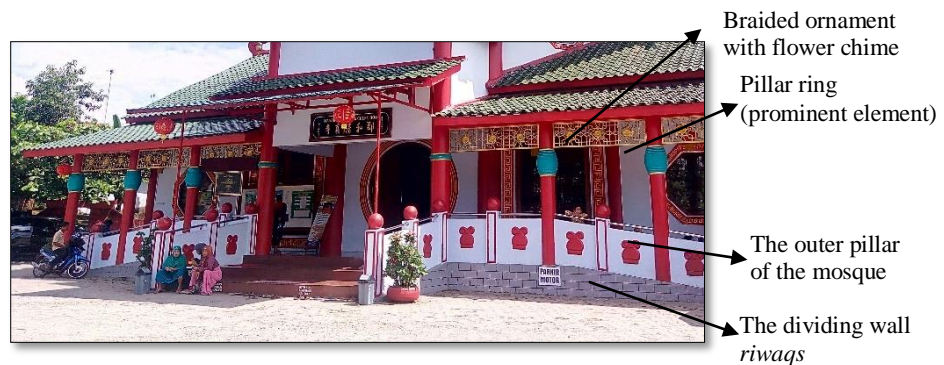
Figure 16. Pillars of the riwaqs boundary of the Cheng Hoo Purbalingga Mosque (Source: Documentation of Imam Ramadhan, 2017)
