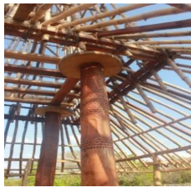
Figure 4. Construction details of top part of pongga bokolo, the circular disc is named lele
