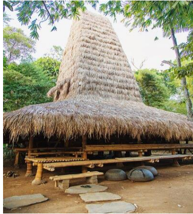
Figure 2: Uma Sumba. Note the stepped platform which structure is independent from the house structure
