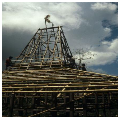
Figure 5. the soaring and sloping roof frame of Uma Sumba
