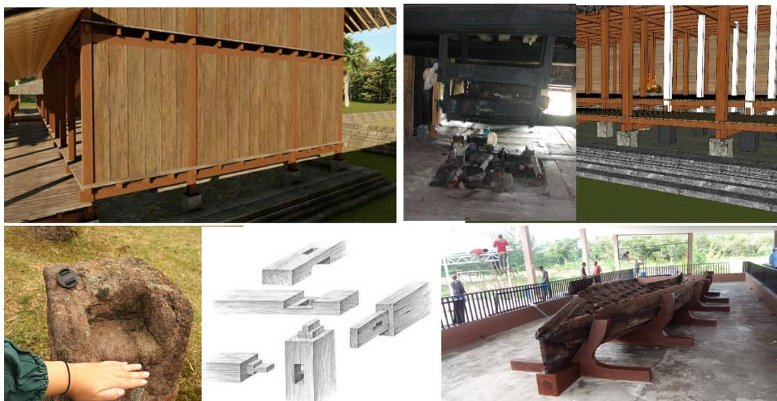
Fig 5. Wooden board, Furnace Analogies (for cold weather), Below : *Umpak* and Square column remain, Wooden Join – *purus*, Boat Wooden Construction[24]
