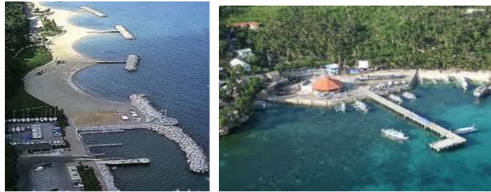
Figure 3. T-shaped Groin and L-shaped Groin
