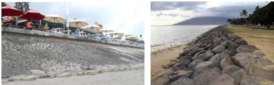
Figure 2. Revetment in General
